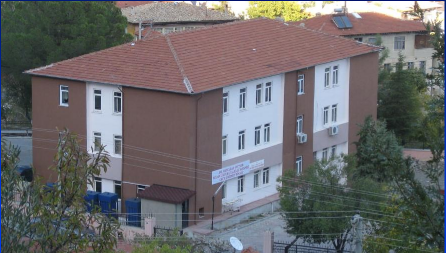
Same building after strengthening
