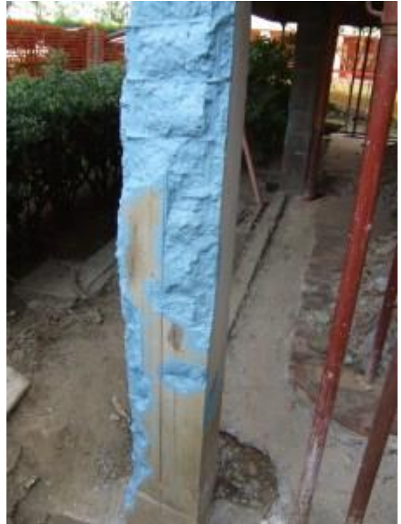
rust removal and passivation of the reinforcing bars
