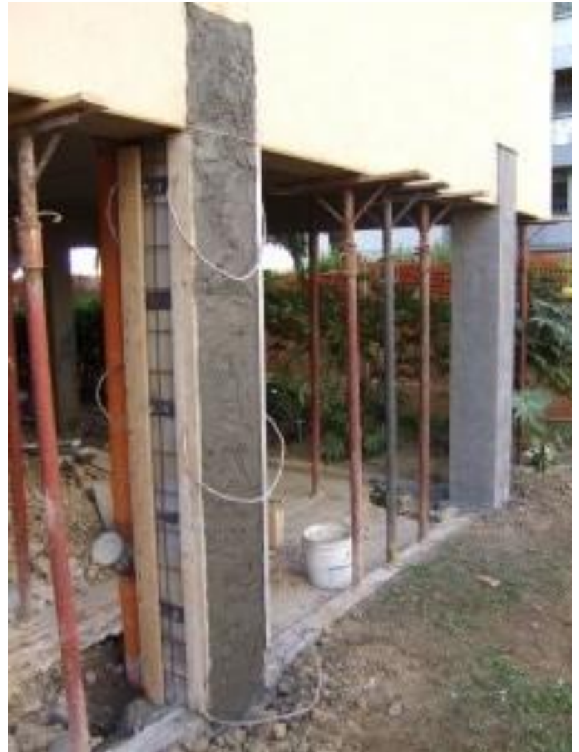
execution of the additional epoxy mortar layer ( s=50 mm)
