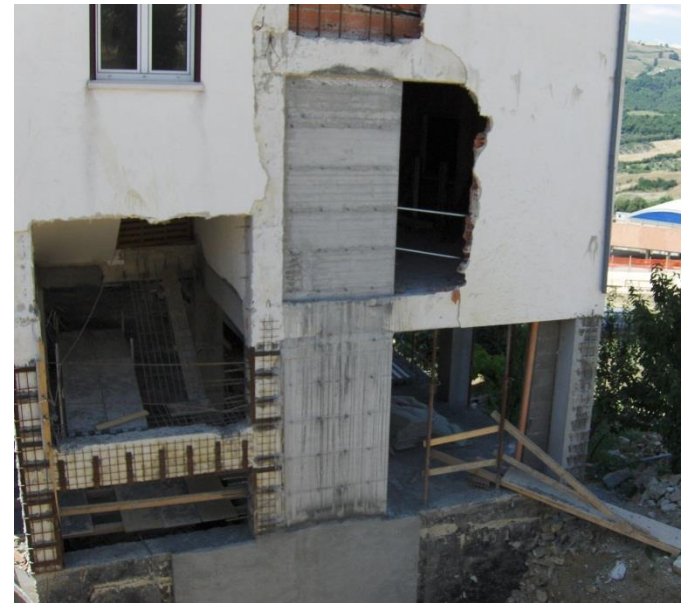
Execution of the shear walls
