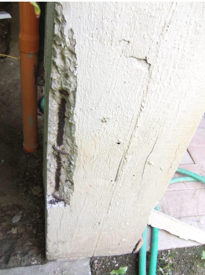
Corroded rebars
