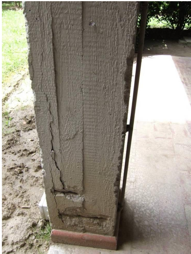
Cracking of concrete cover
