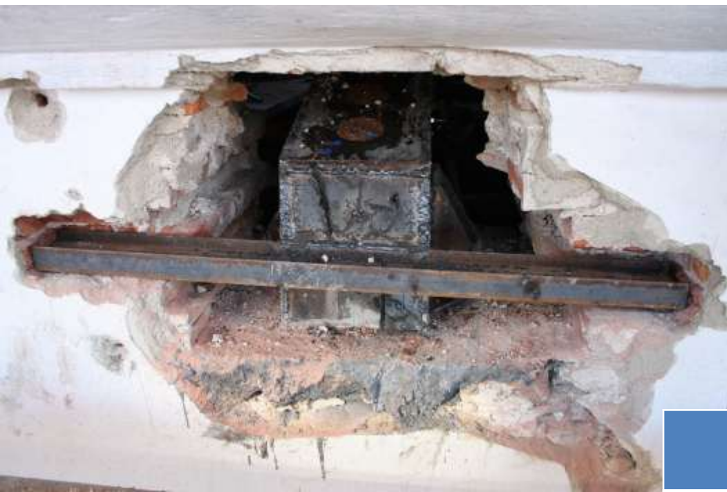
Repair of a damaged head
