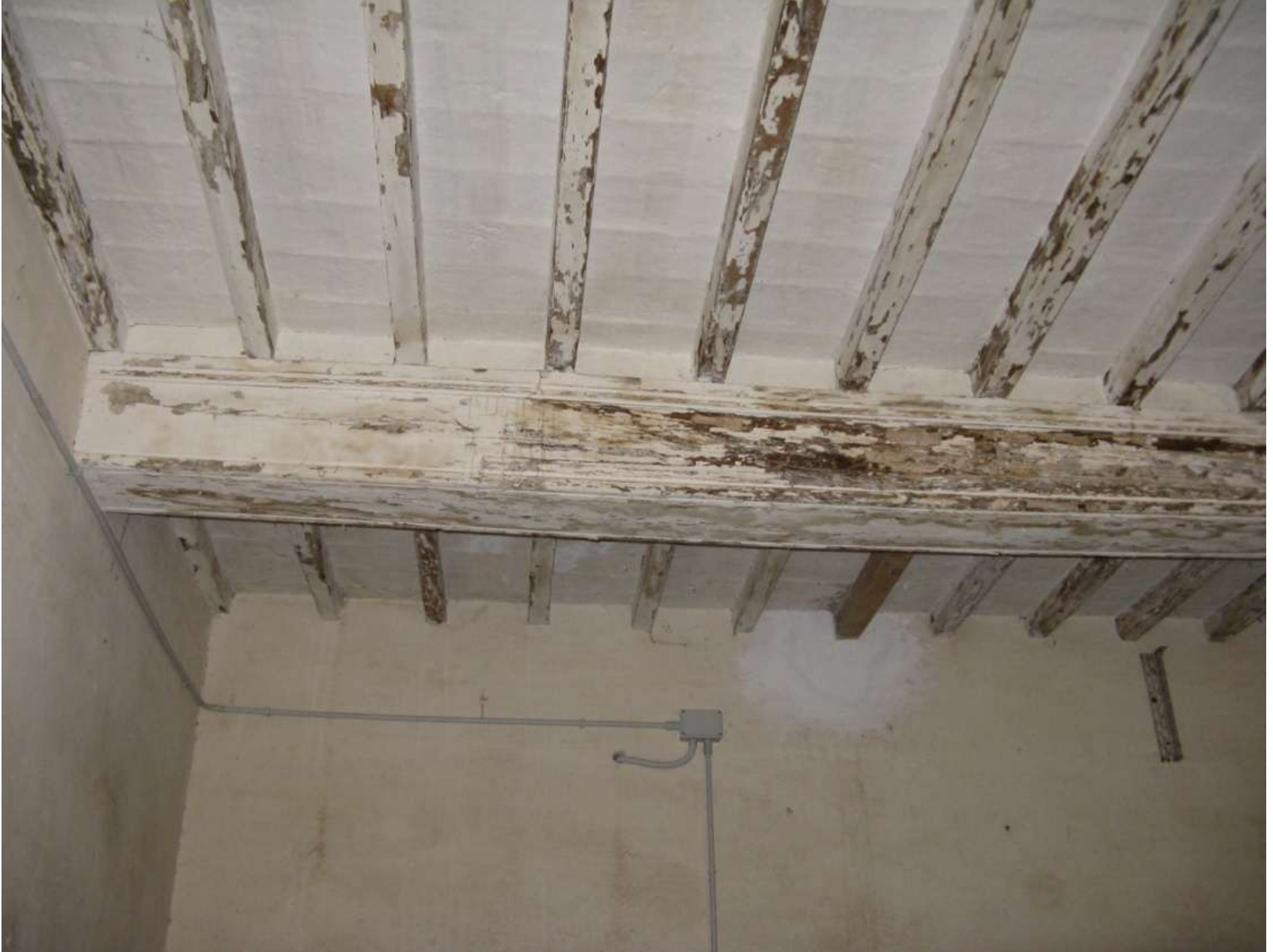
Beam covered with wood plates
