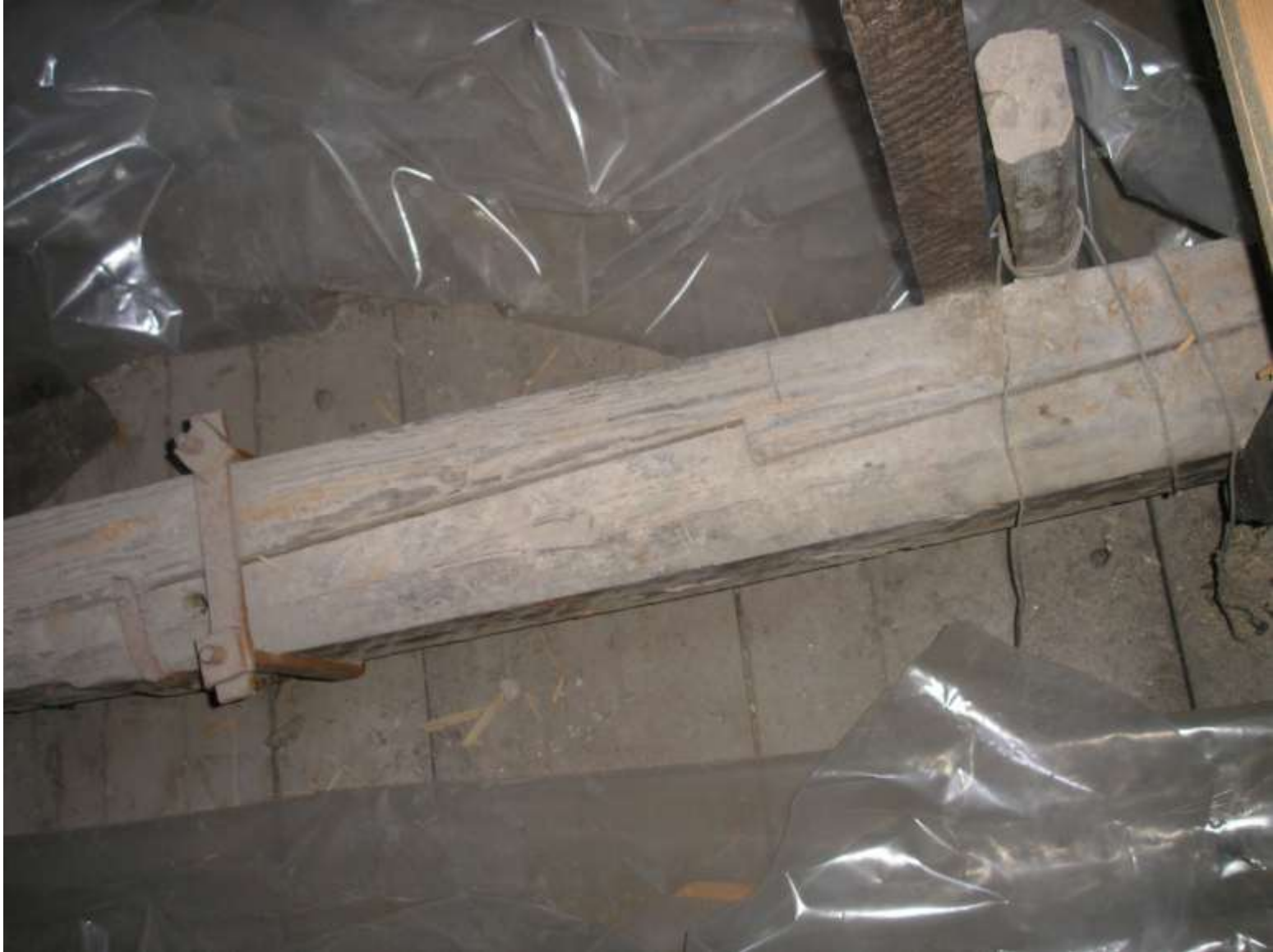
Connection of the truss tie - Jupiter dart
