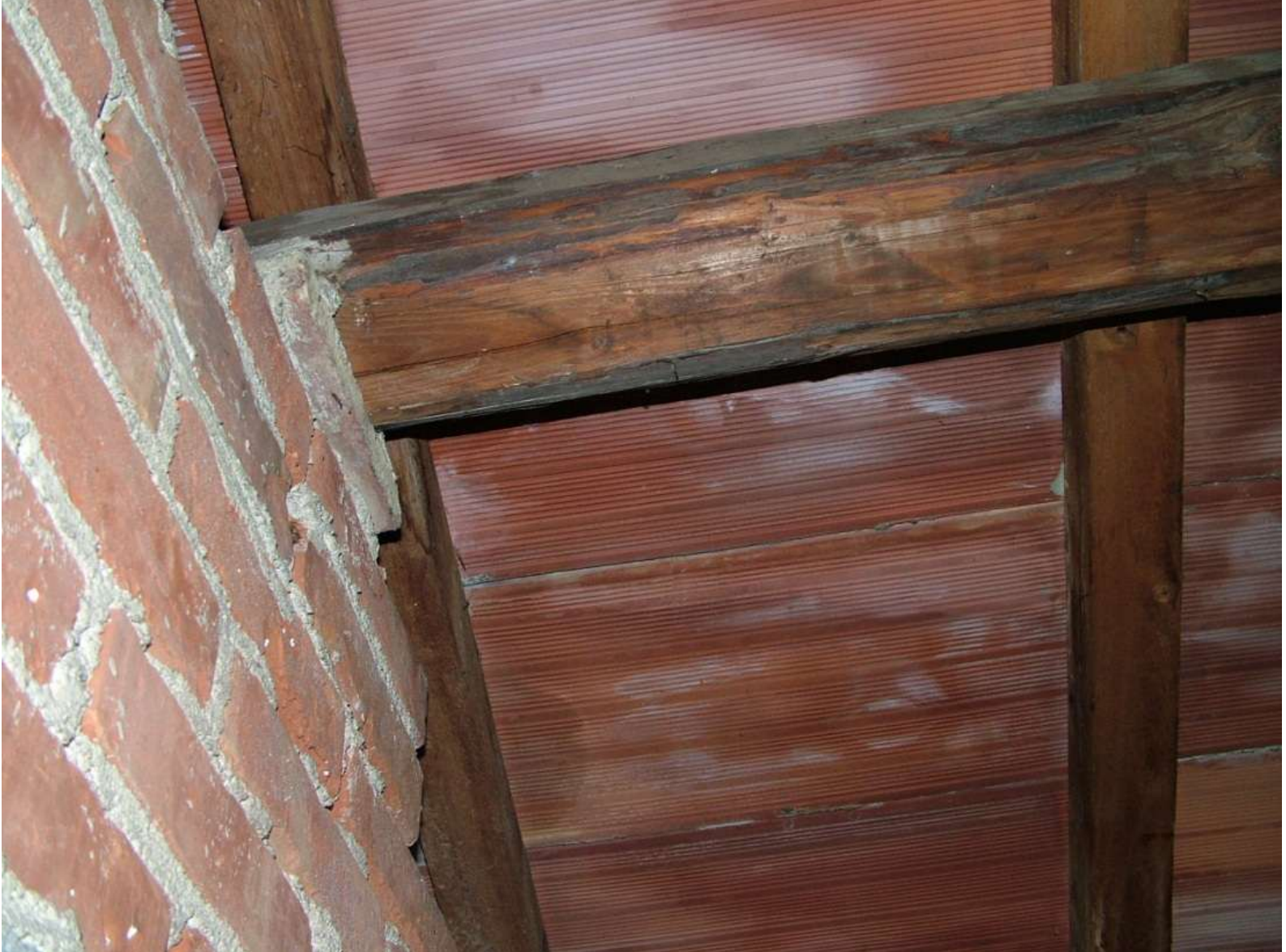
Crack pattern in a beam
