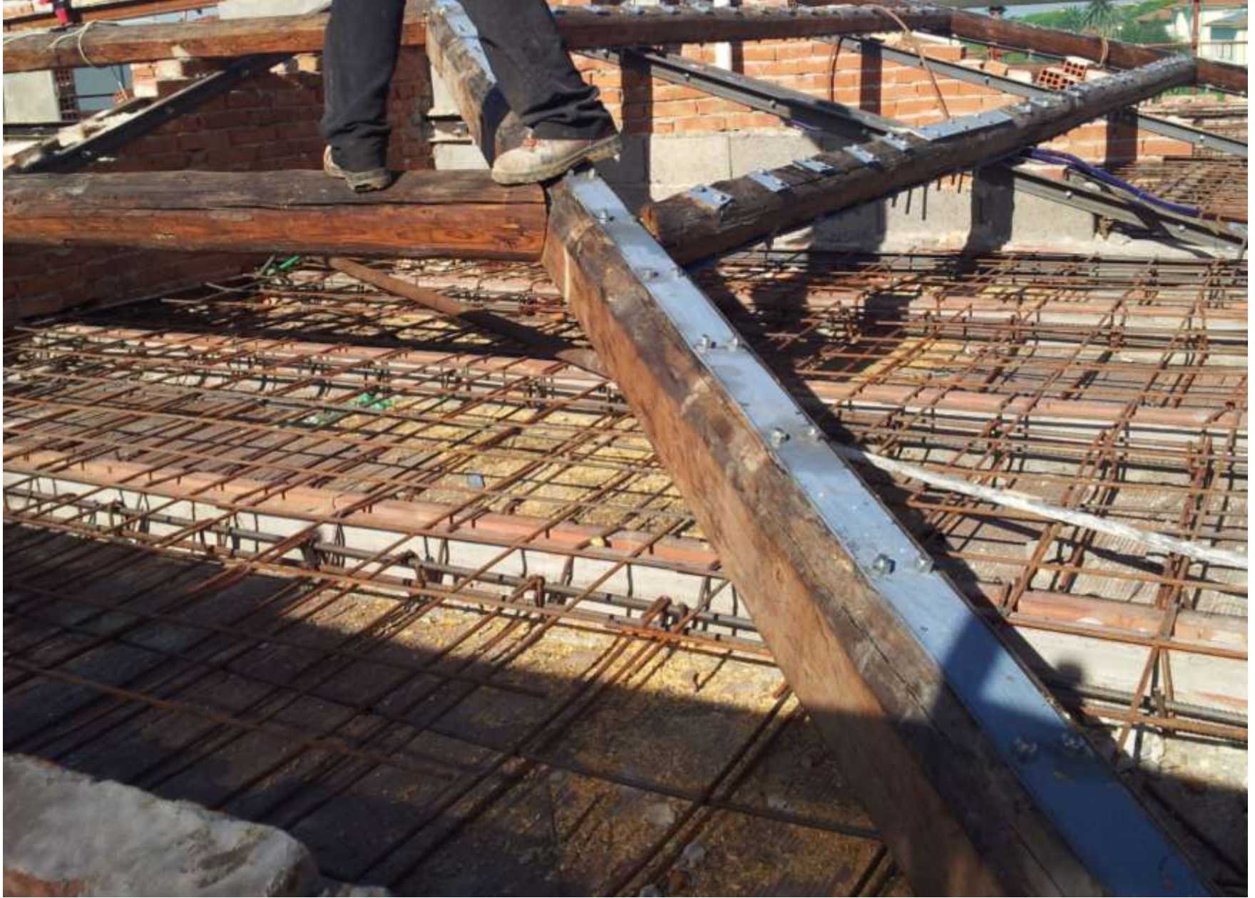
Strengthening of the main beams
