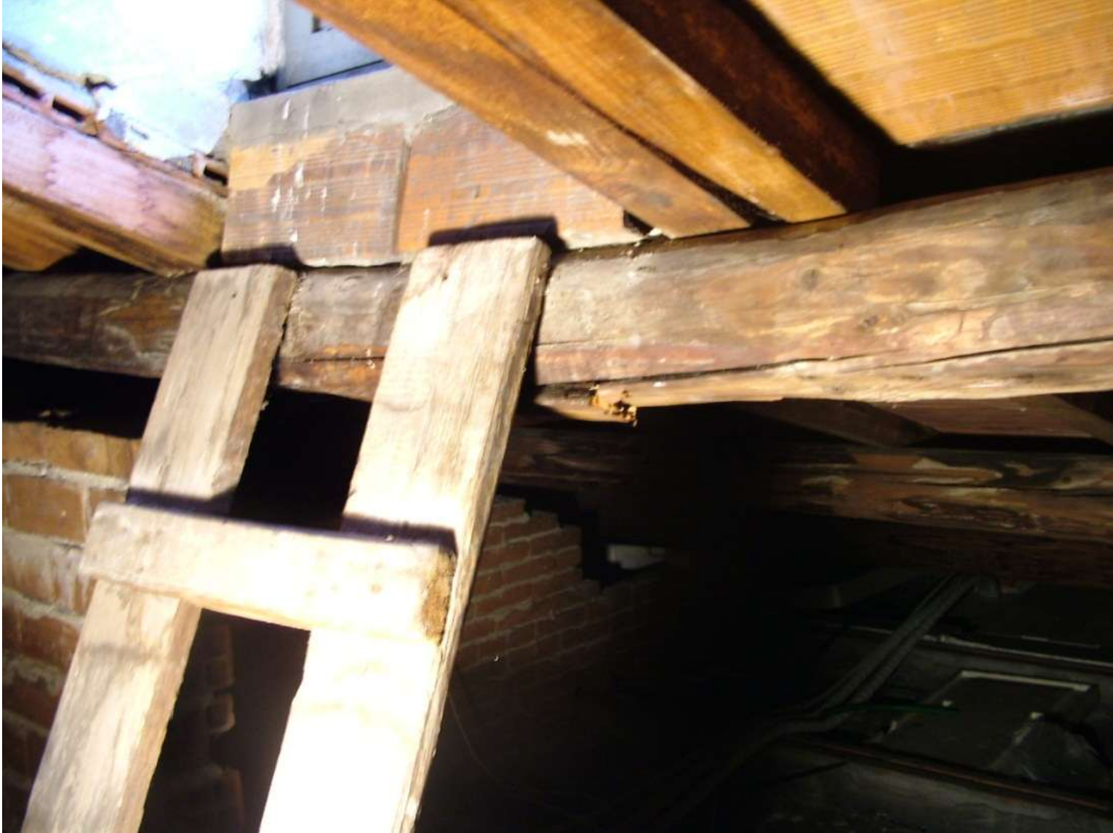
Cracked beam
