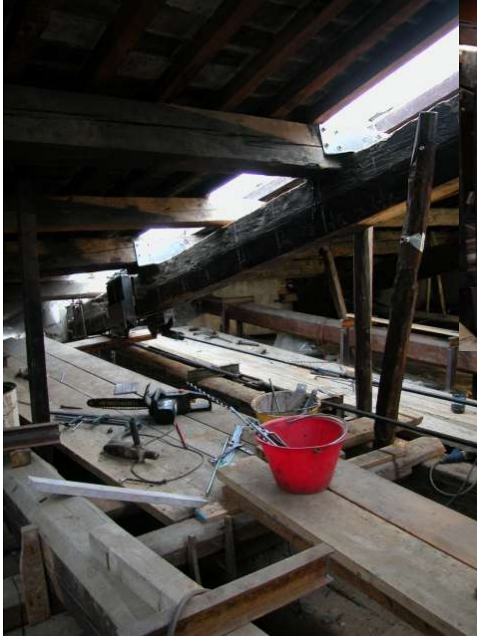
Repair of the truss and temporary chain
