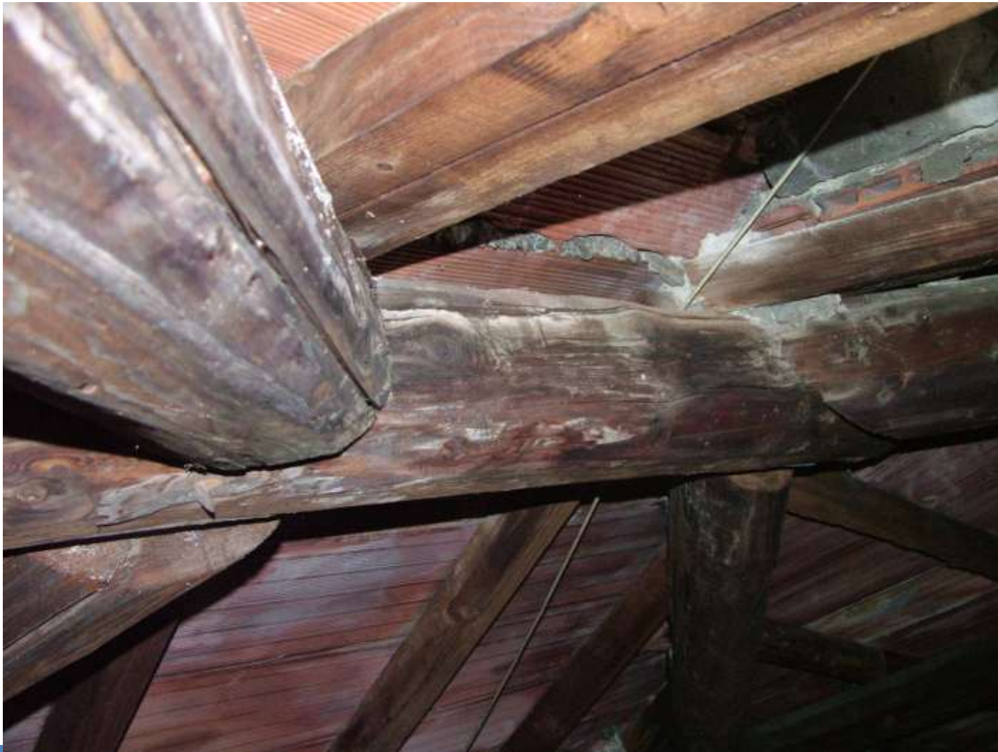
Cracked beam
