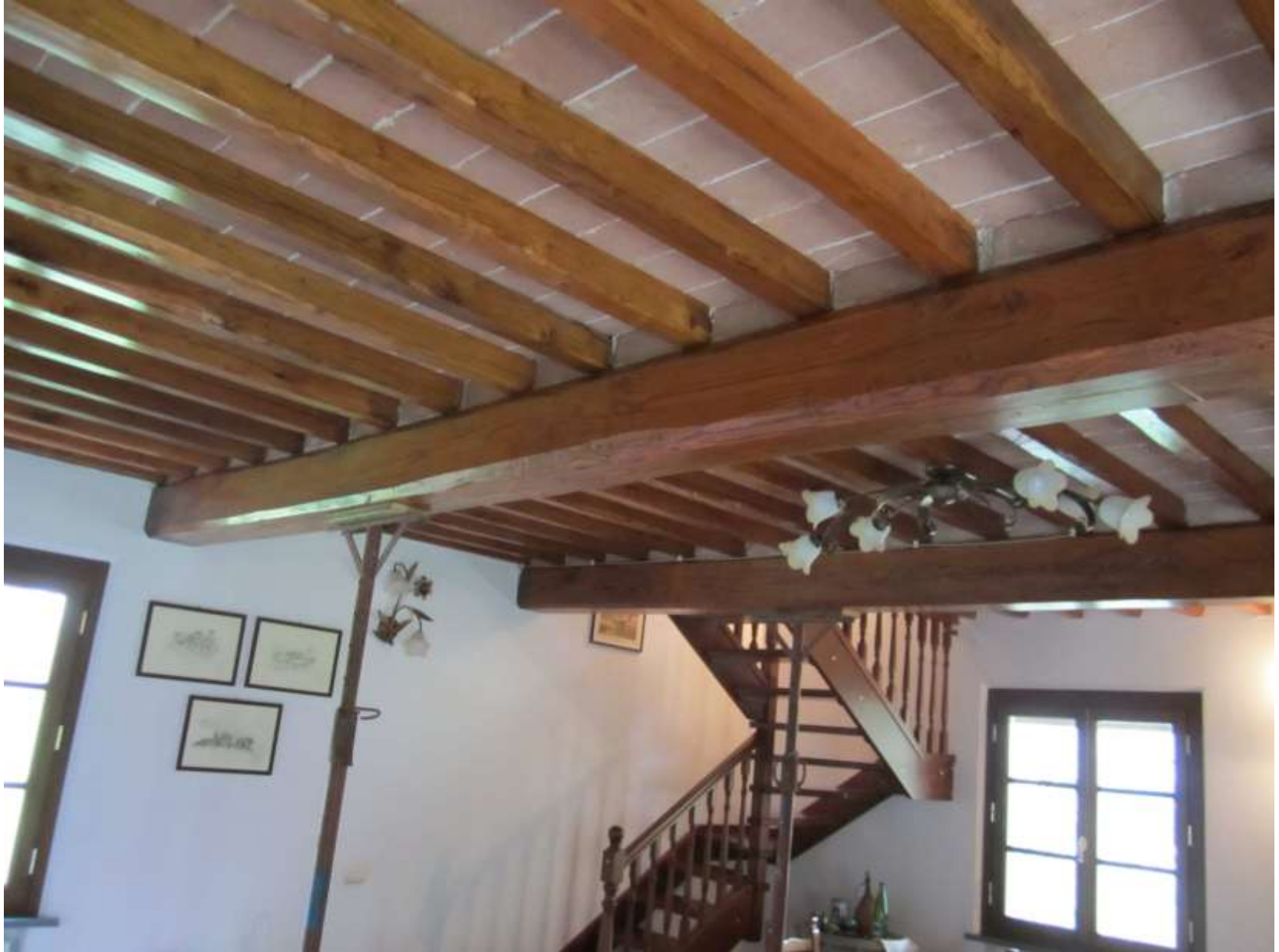
Beams supported with pack props
