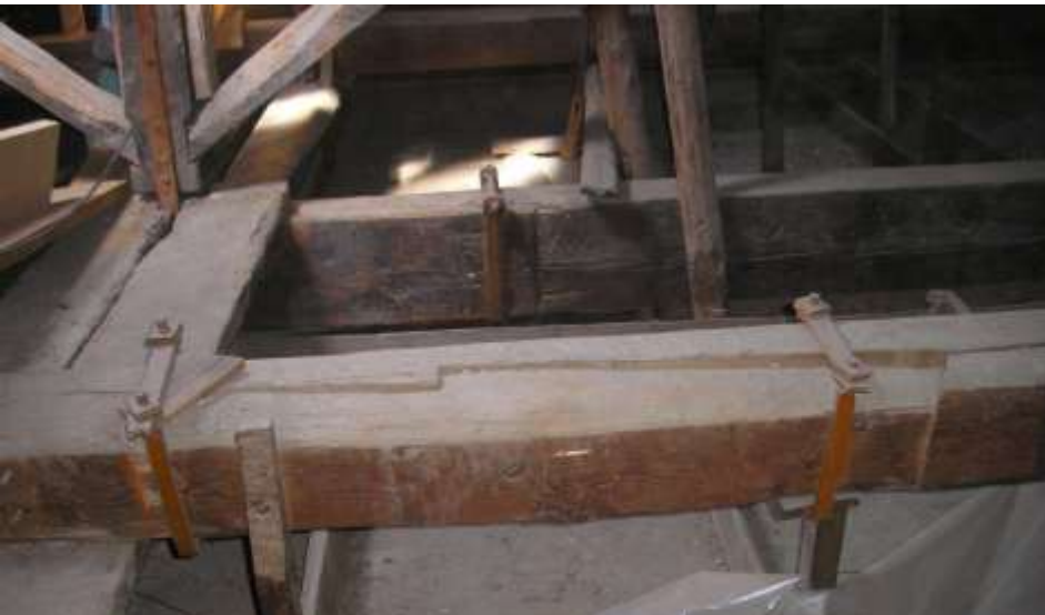
Connection of the truss tie - Jupiter dart
