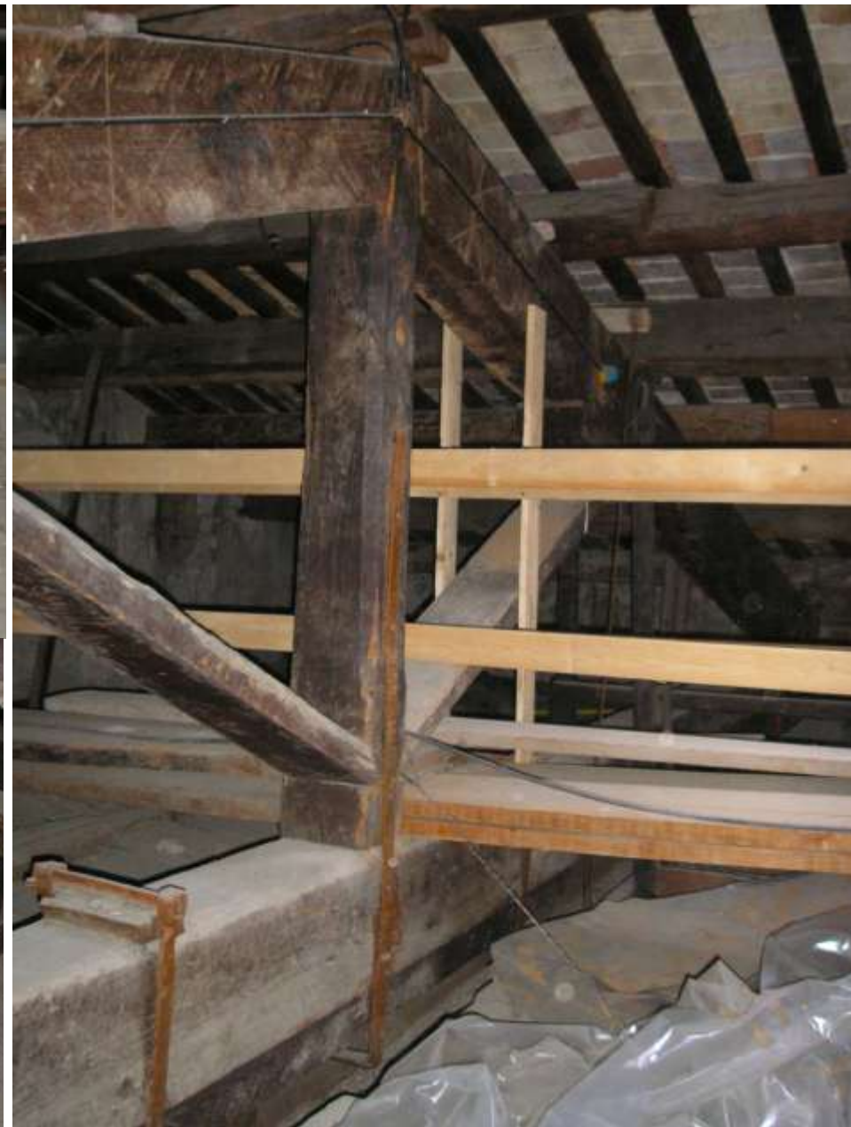
Suspension of the cieling
