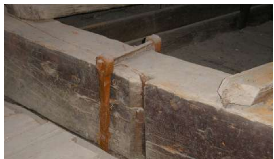
Connection of the truss tie - Jupiter dart
