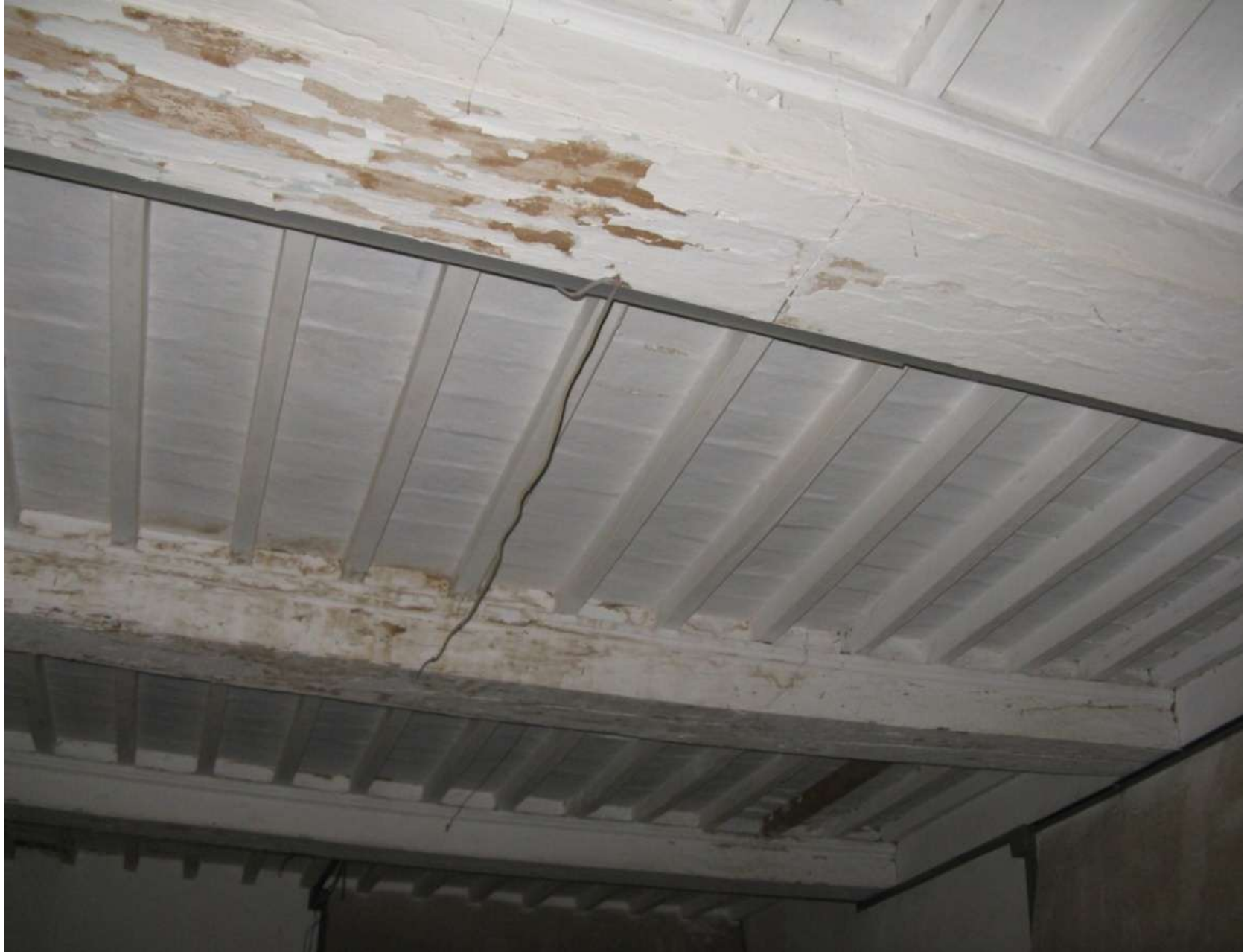
General view of the floor
